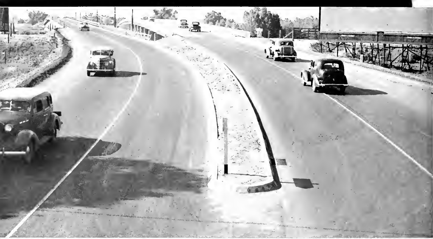
View of divided road at northerly approach to new and old bridges over Kern River on State Route 142
